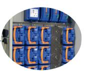
Transparent fuse way shield padlocked in place.
